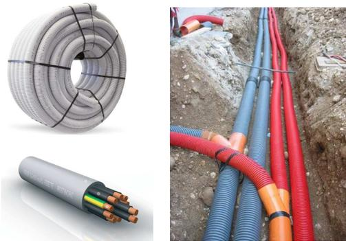
The electric network, required to transport the energy from the generator to the various user, are designed and manufactured employing electrical cables with double insulation, installed in underground pipes or on a appropriate poles depending on the location and type of user.
