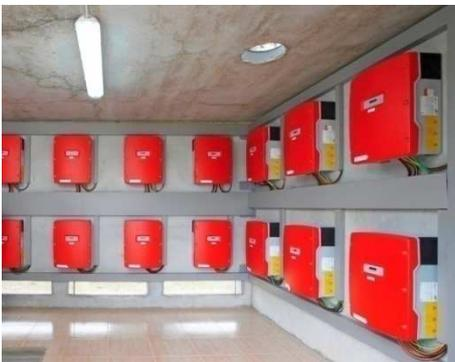
The inverters allow a smart power management of the energy produced, which can be stored in the battery pack or fed into the grid. It is possible to operate with several values of voltage and frequency, with two kinds of distribution (single phase or three phase).
